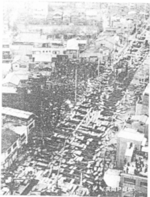
Fig. 1 Spot of gas explosion accident.
