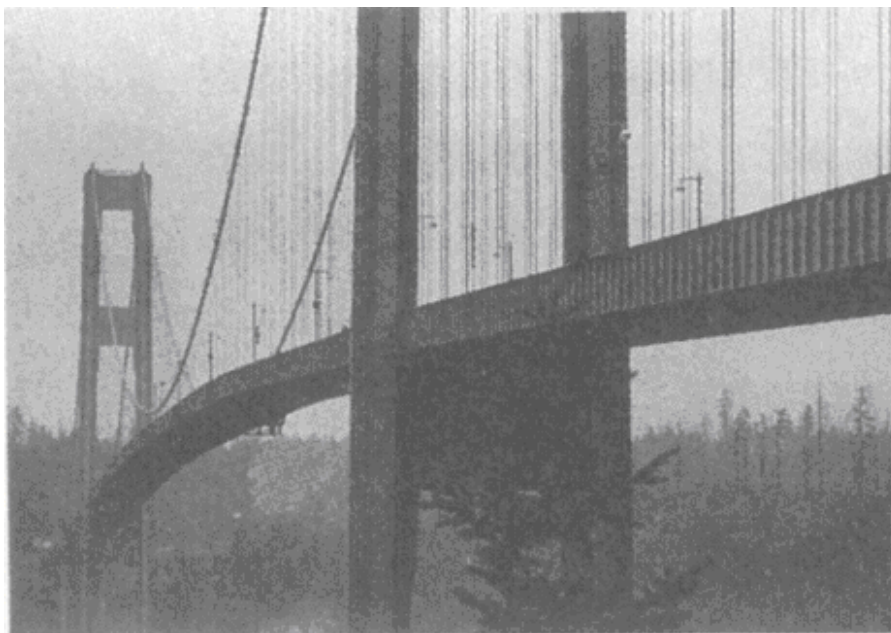
Photo 3. The former Tacoma Bridge (its bridge girder has a flat H form) [1]
