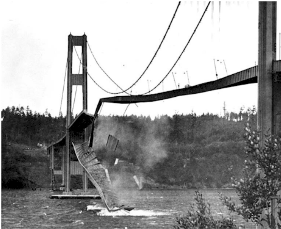
University of Washington Libraries, Special Collections, FAR017 Photo 2. Breakdown of Tacoma Narrows Bridge [1]
