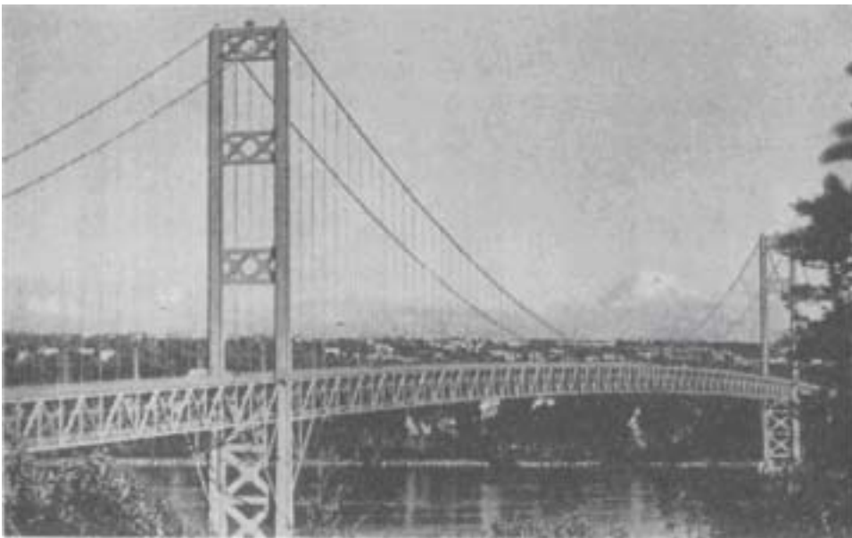
Photo 4. New Tacoma Narrows Bridge (with Open Trusses) [1]
